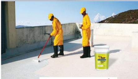
Dr. FIXIT Pre-monsoon repairs
